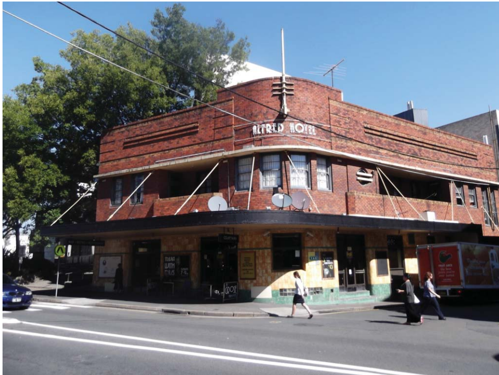
Figure 3 View from Missenden Road
